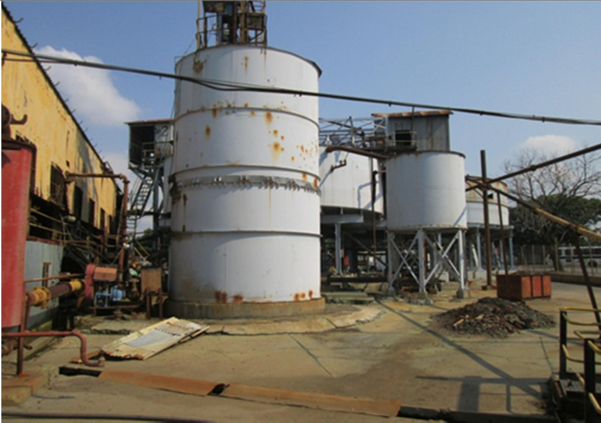
The Filtration Area
