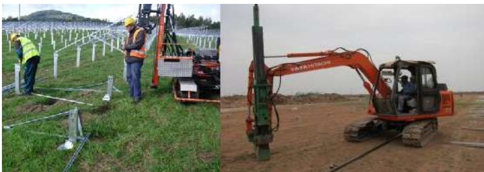
Figure 7: Construction of PV plant (Image from www.aceinfra.com and www.kaska.eu )
