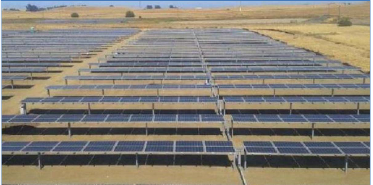
Figure 1: Example of a Photo Voltaic Solar Power Facility.
