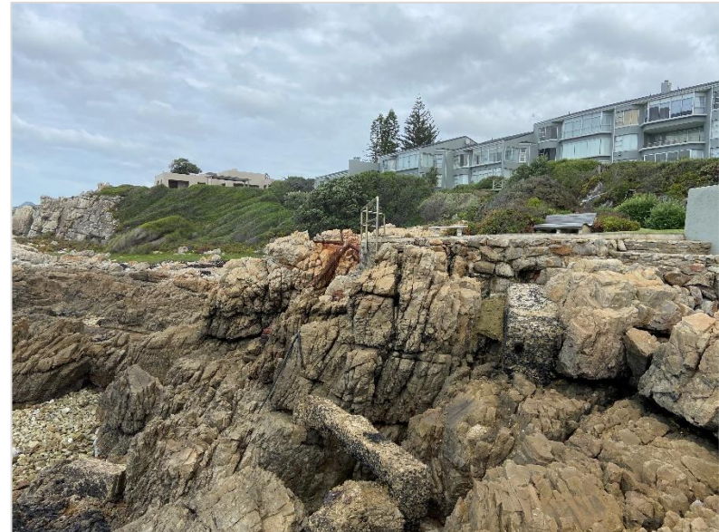
Figure 16: Area below Bay View Apartments where and elevated section is needed
