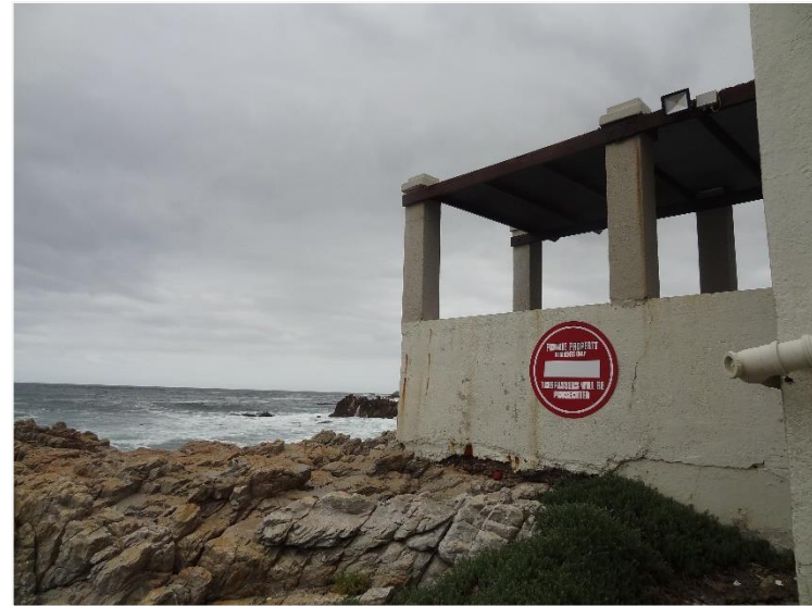
Figure 30: Path to go around building at Bayview pool
