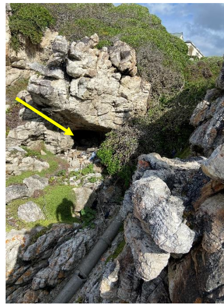
Figure 8: Gully with stormwater pipe where access was proposed for Alternative 1, also showing small cave used by vagrants (yellow arrow)
