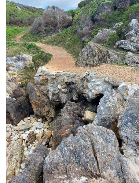
Figure 34: Existing Cliff path in steeper areas with natural stone finish
