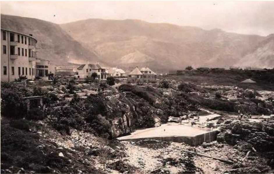
Figure 25: Historical photo of old Bayview Hotel after it was rebuilt in the 1940's
