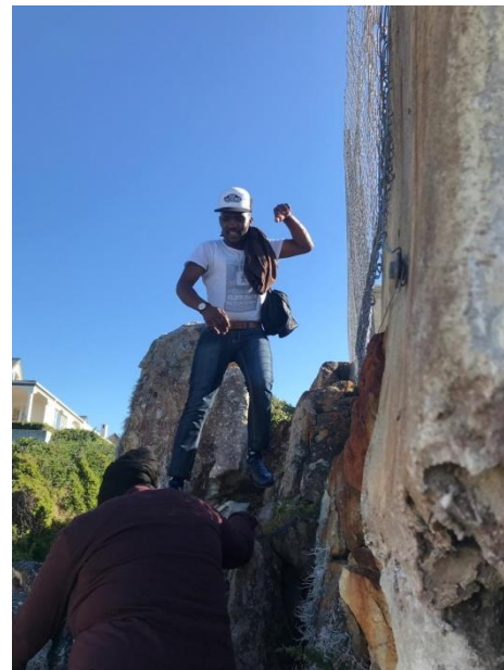
Figure 6: Current difficult access against fence line at Erf 12257
