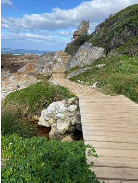
Figure 35: Boardwalk crossings on existing Cliff path. Wetland and stream areas on connection path to have similar structures for minimal impact on these features.
