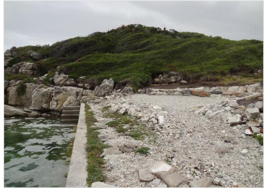
Figure 22: Tidal pool and pebbles / gravel. An elevated section along the rocks is proposed to the back left in the picture with a flat concrete path on the right edge of the pool.
