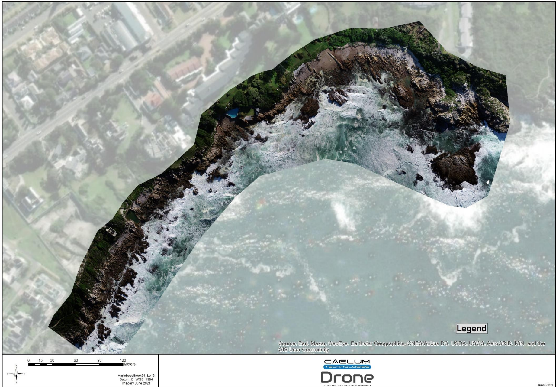
Figure 40: Birdseye view of Poole's Bay area, photo taken at low tide - note that the Island is not accessible (Photo: Caelum technologies, 2021)
