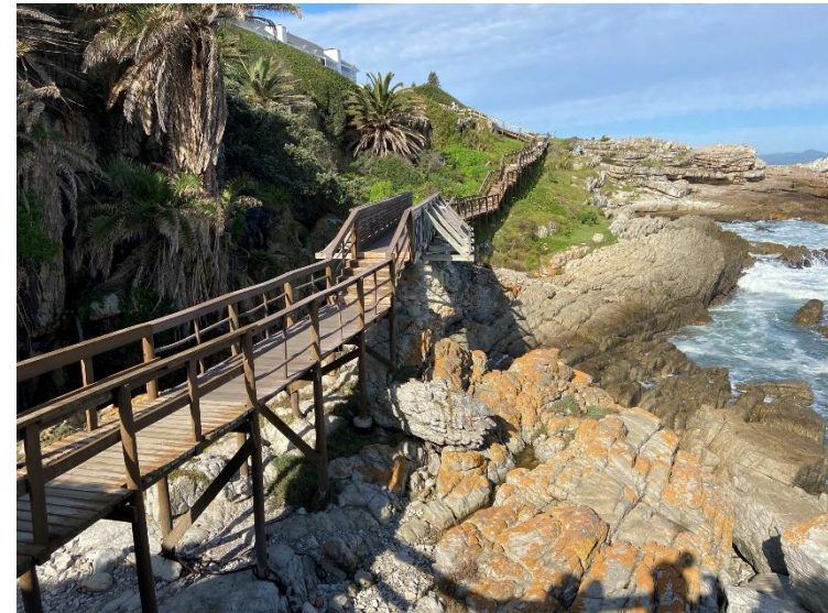
Figure 36: Elevated bridge on existing Cliff path. Bridge structures for connection path is proposed to be in concrete to withstand rough sea conditions
