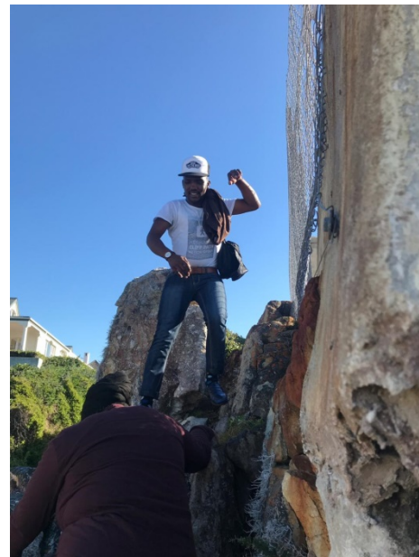
Figure 6: Difficult access against fence line at Erf 12257
