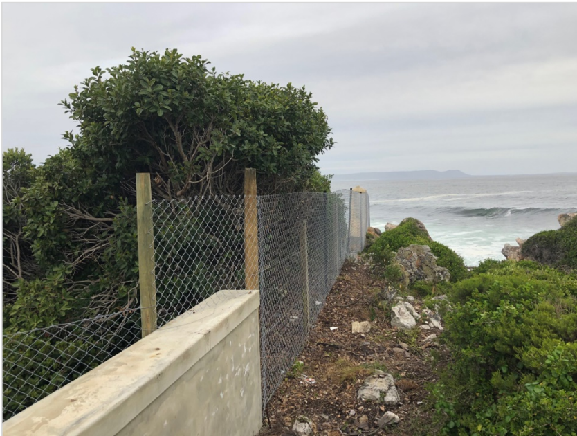
Figure 3: Western entry to proposed connection path, which is currently hindered due to a fence erected by the owner of Erf 12257
