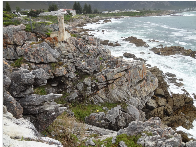
Figure 4: View of the area where fence was put up. The path would have to go down and around the pillar to the right in the picture through dowelling into the rock.
