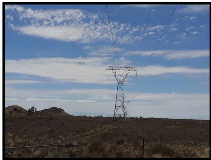
Photo 3: This photo shows a typical OHPL comprising lattice structures.
