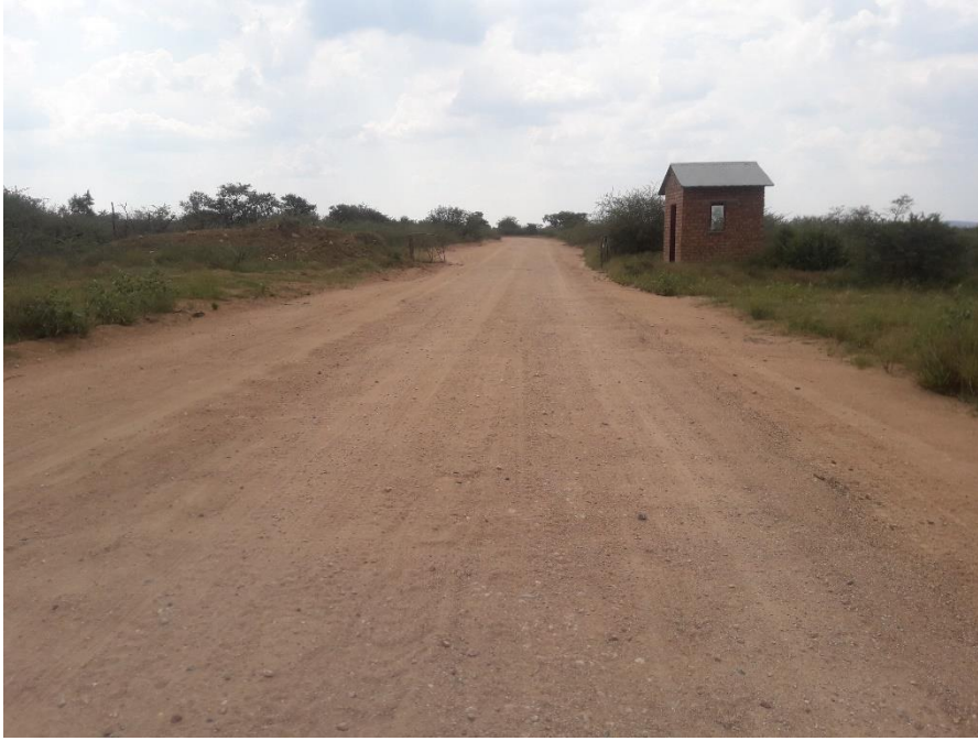
Figure 6: Access road used on site, maintained by Sand Hawks
