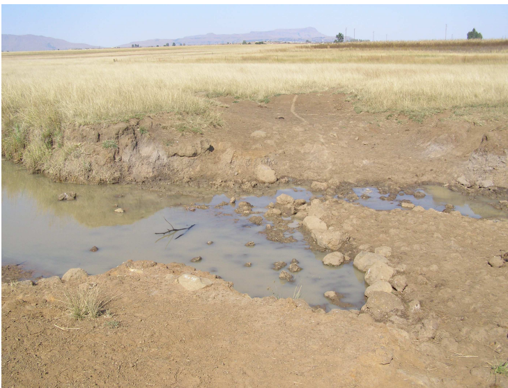
Photo 2: Wetland A showing erosion at road crossing.
