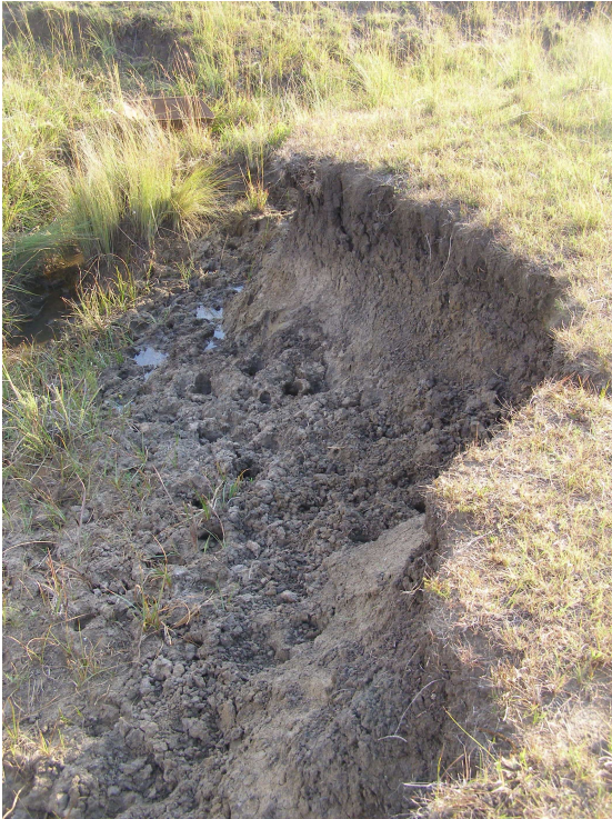
Photo 1: Wetland A showing erosion of river bank as a result of cattle trampling.
