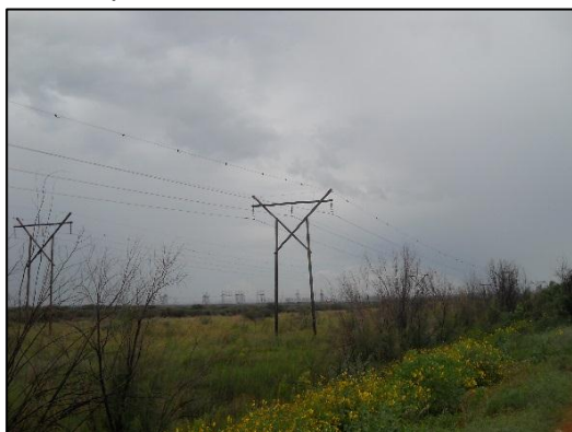
Figure 28: Power lines near the impoundment.
