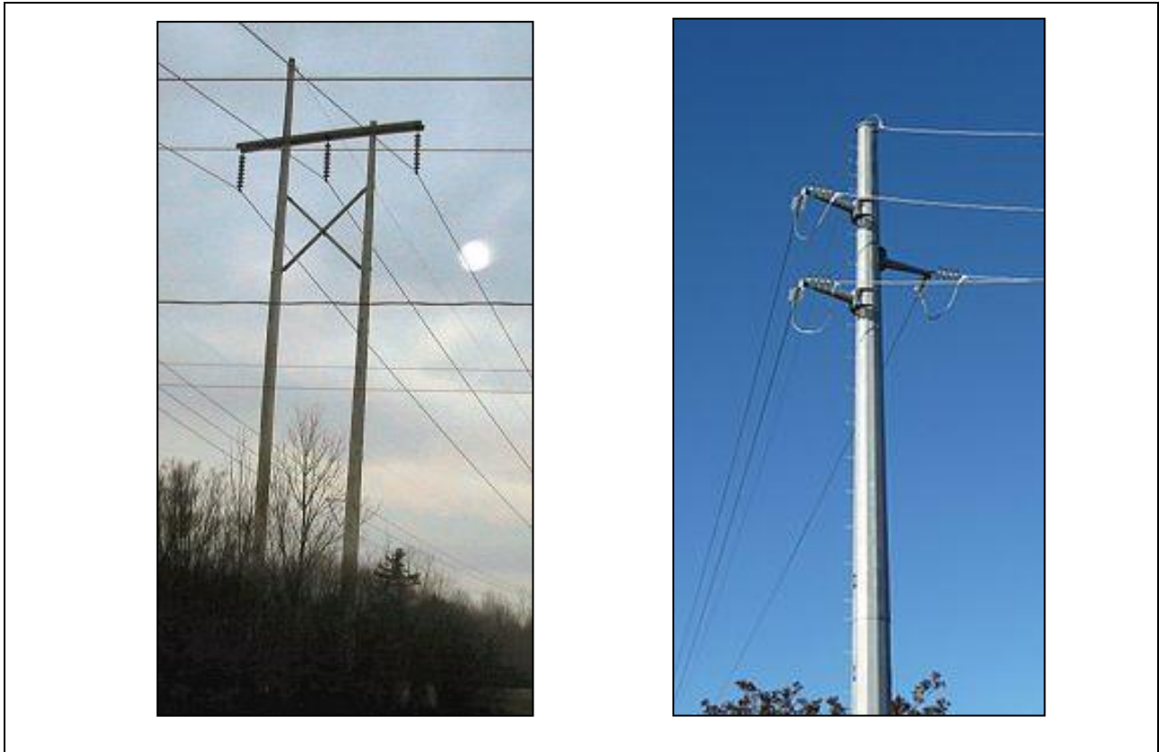
Examples of H-poles that will be used during the construction of the proposed transmission line.
