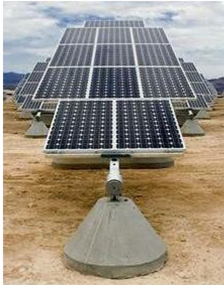
Figure 16: Precast footing on tilted single axis tracker (image: ens-newswire.com)
