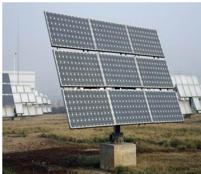
Figure 15: Shuttered foundation with double axis tracking (image: www.tradekorea.com )
