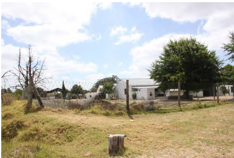
Figure 8: The existing sheds on site.
