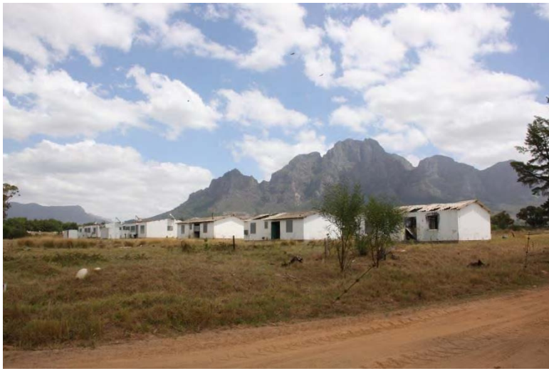
Figure 4: The dilapidated and vacant farm worker's cottages.
