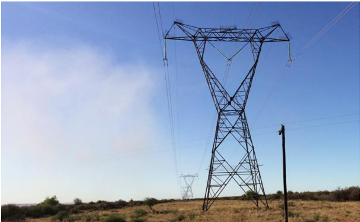
Figure 6: View northwest from Photo 6 location of the existing Eskom power line under which the proposed 132kV power line will be routed.
