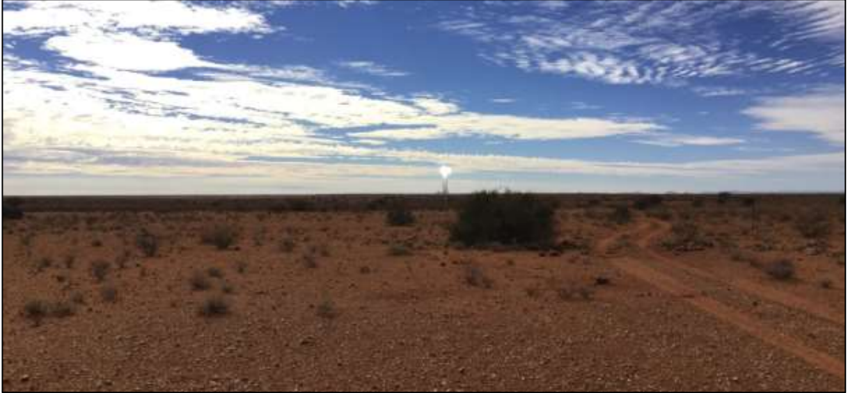
Survey Point 9 photograph taken towards the east of the Khi Solar One CSP Tower as seen from the proposed development footprint.
