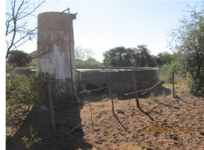
Figure 9: One of two water reservoirs connected to borehole / solar pump, located within north-eastern portion of study-site.
