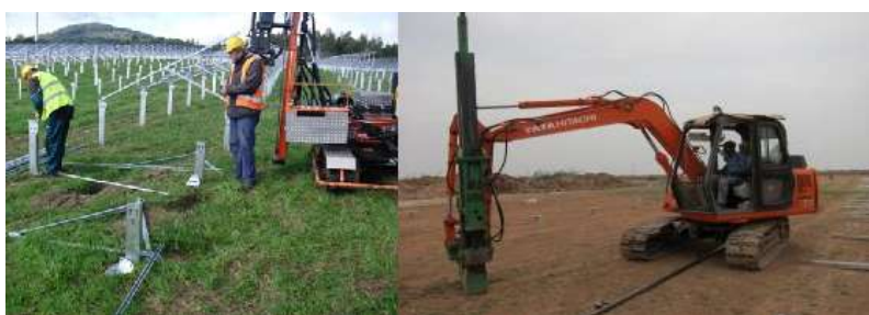
Figure 9: Installation of frame foundation (Image from www.aceinfra.com and www.kaska.eu )
