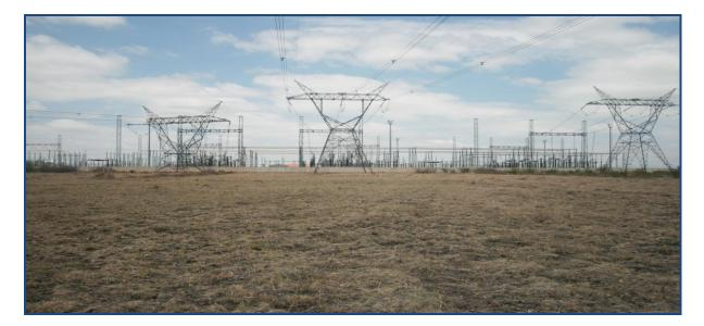
Figure 3: Bighorn – Marang and Medupi-Marang 400kV power lines feeding into Marang MTS
