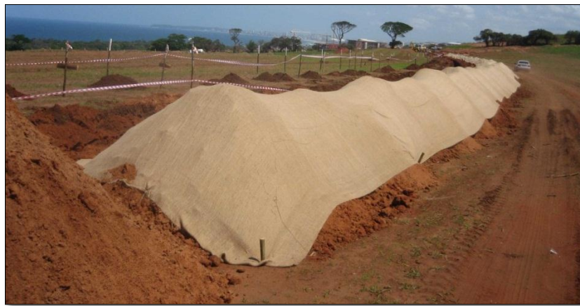
Figure 43: Soil stockpiles covered with hessian sheets
