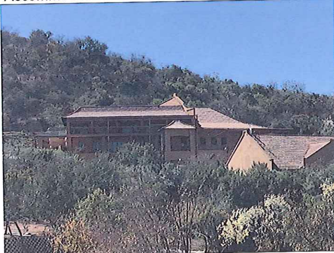
Restaurant building at back (including restaurant, spa, small restaurant or break-away rooms) and Accommodation Block 2 – 12 en-suite rooms
