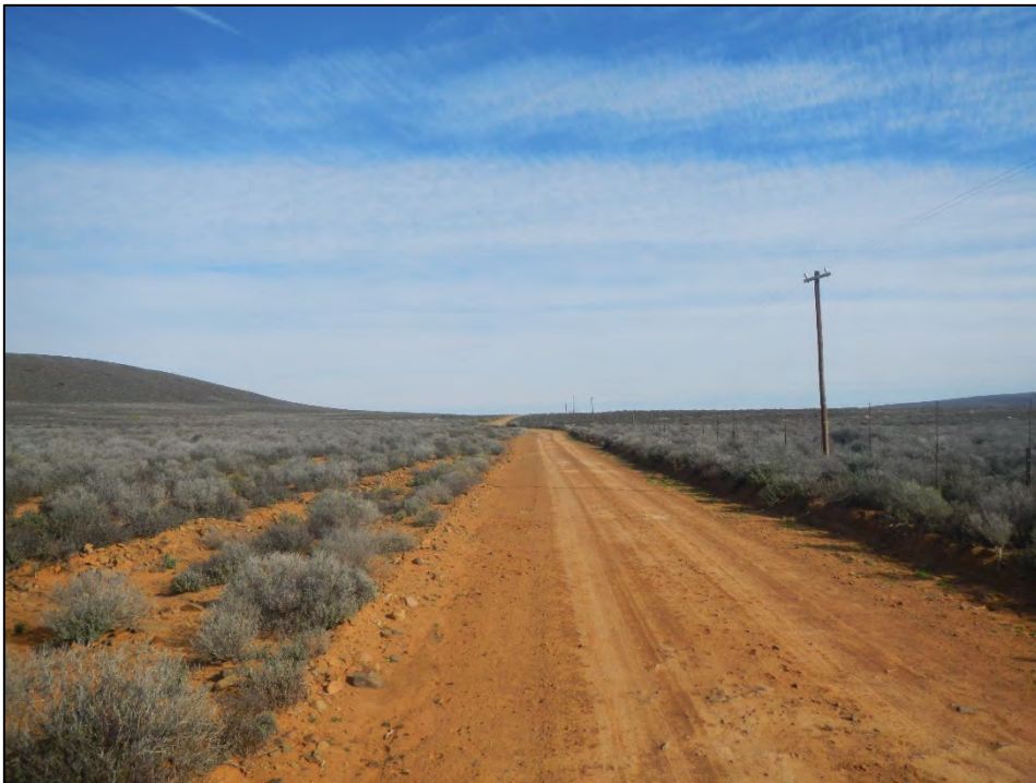
Figure 17: Typical view of telephone lines found within the study area
