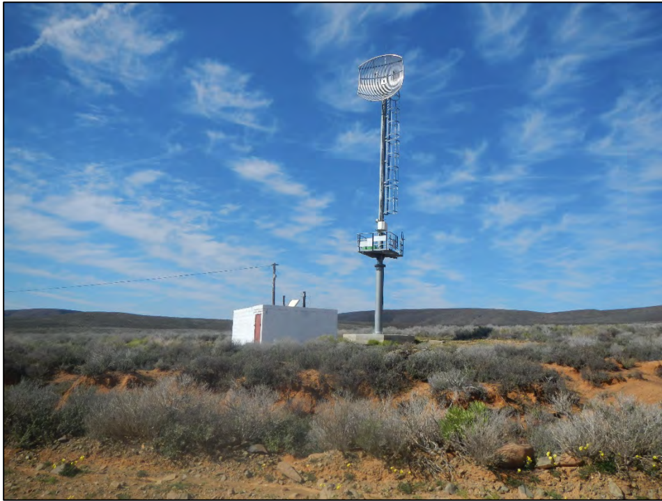
Figure 20: View of a relatively tall tower found within the study area
