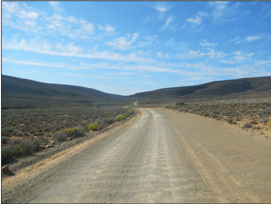
Figure 21: Typical view of the R356 Regional Route
