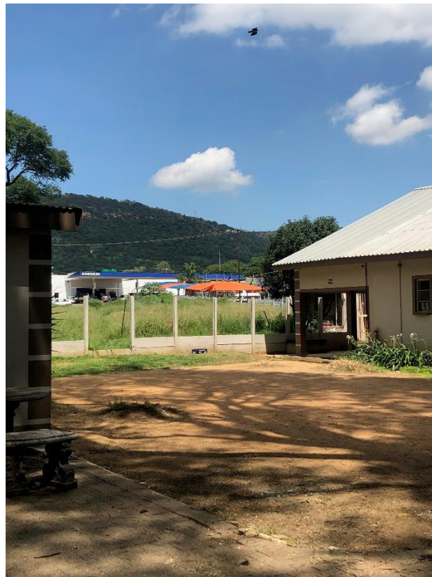
View from property standing at the house looking south west towards southern property boundary, R565 and Engen Filling Station
