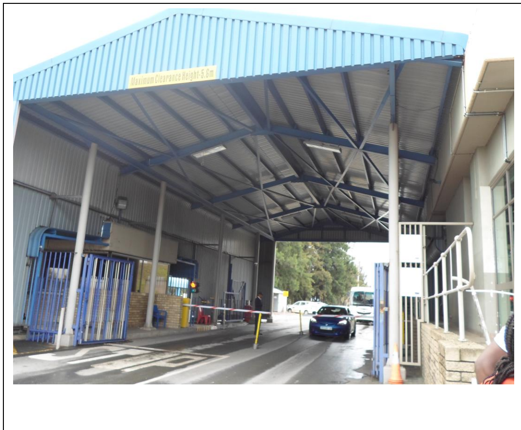
Figure 1: A2 Site notices placed at the Lethabo Power Station entrance gate
