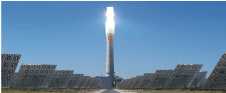
Figure 2: The Central Tower – Gemasolar
