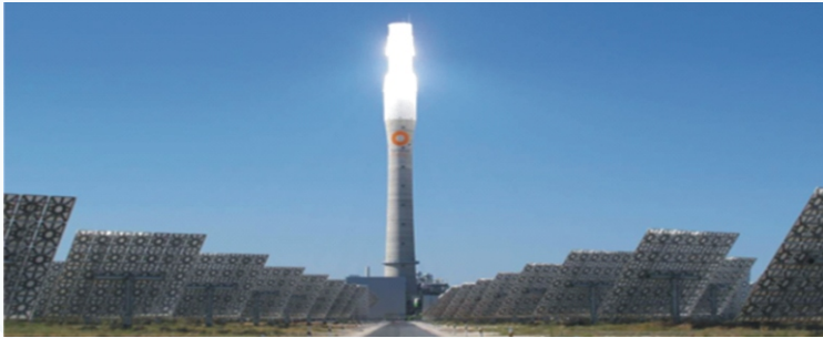
Figure 2: The Central Tower – Gemasolar
