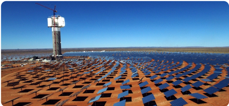
Abengoa's Khi Solar One STE tower plant under construction near Upington.
