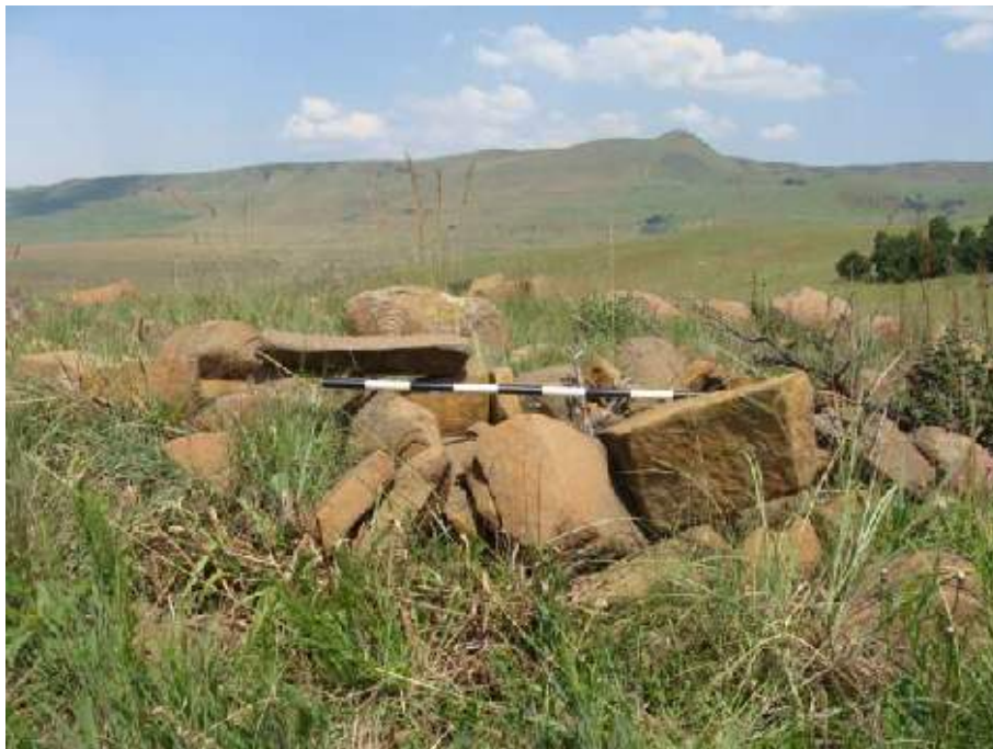
Figure 7 Site no. 2, a defensive wall.
