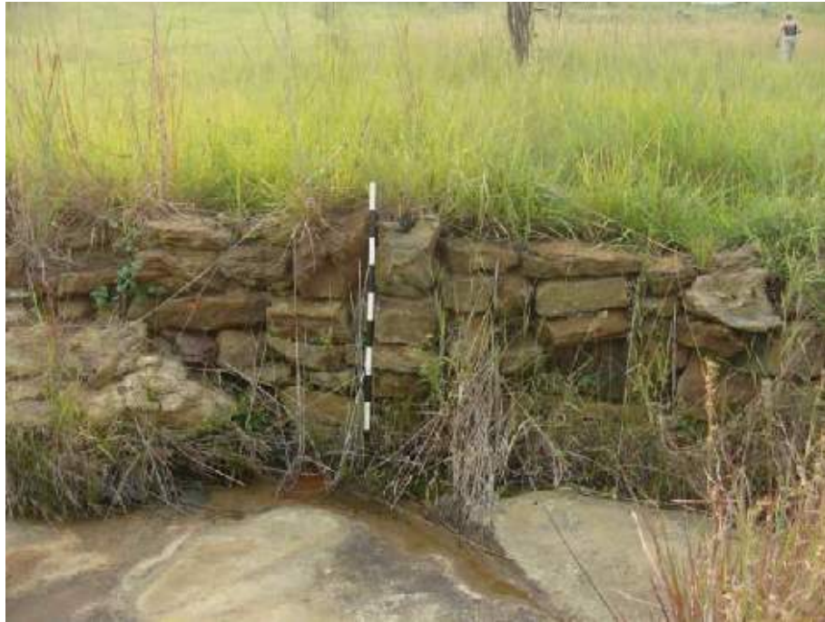
Figure 20 Possible dam wall at site no. 13.
