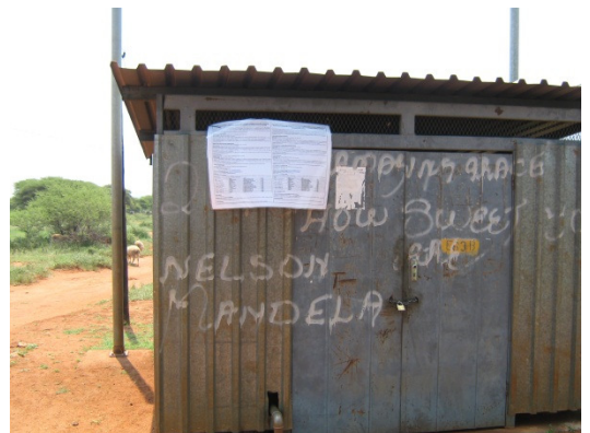
Photo 38: Magalane pump station
