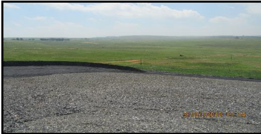
Figure 3: Photo showing the terrain across which the proposed conveyor is to traverse (taken from the top of the Discard Dump)
