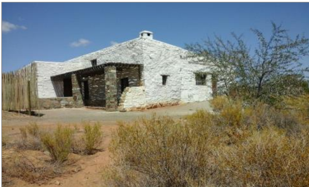
Photograph 3 - Man-made infrastructures with suitable characteristics for roosting of bat species.
