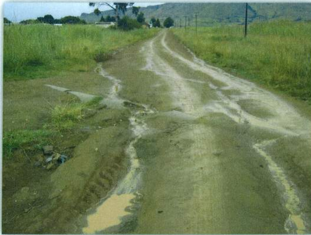
PHOTO 11: Dirt Road from Dirkiesdorp to Proposed Mine (Photo 1)
