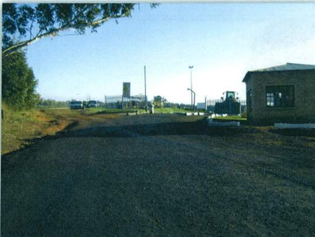
PHOTO 4: Entrance Road to Railway Siding (Photo 1)
