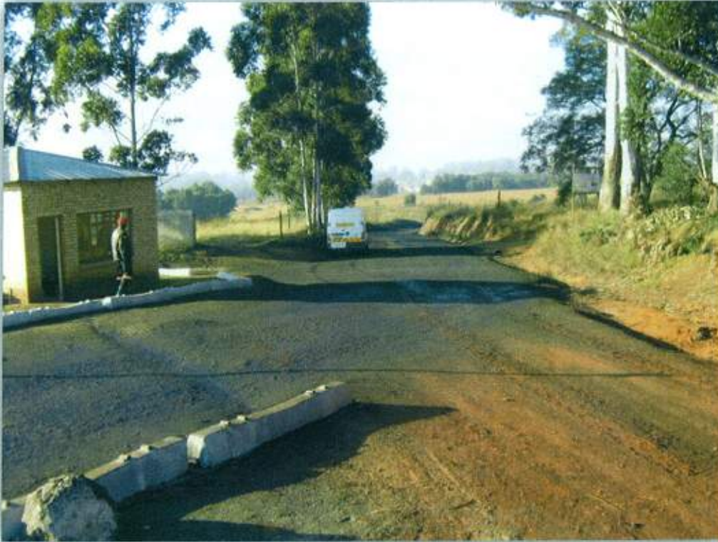
PHOTO 5: Entrance Road to Railway Siding (Photo 2)
