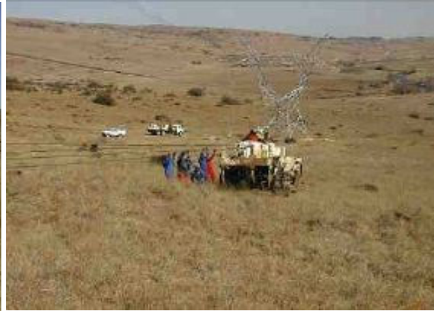
Stringing pilot cable with pilot tractor
