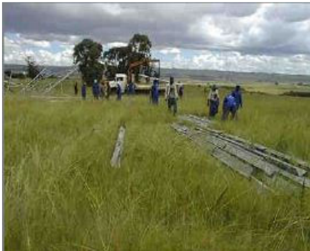
Steel delivered for assembly
