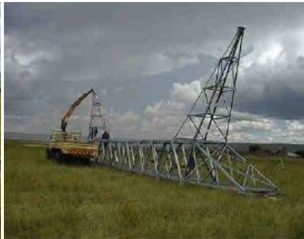
Assembled pylon
