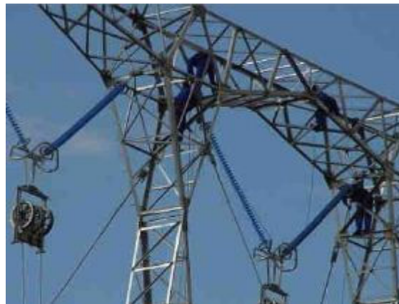
Using pulleys to hoist cable
