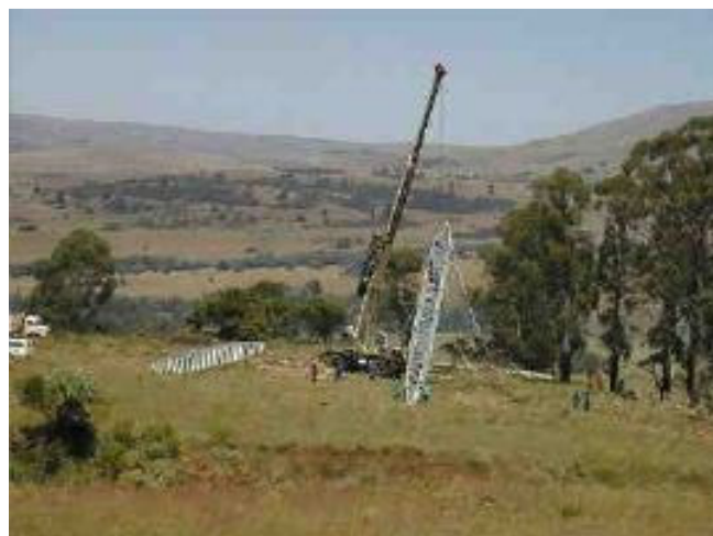
Raising the pylon
