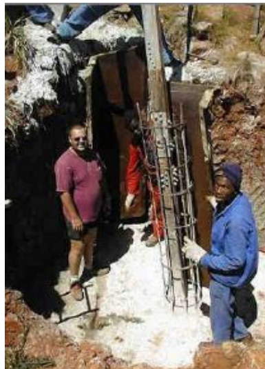
Foundation steelwork
