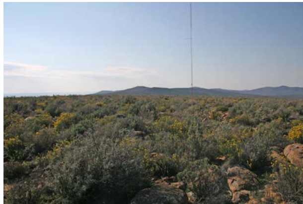
Figure D6: Mountain crest with one of the four communication towers.
