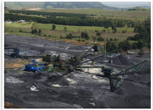
Photograph example of stockpile infrastructure, Kiepersol Colliery, Piet Retief
