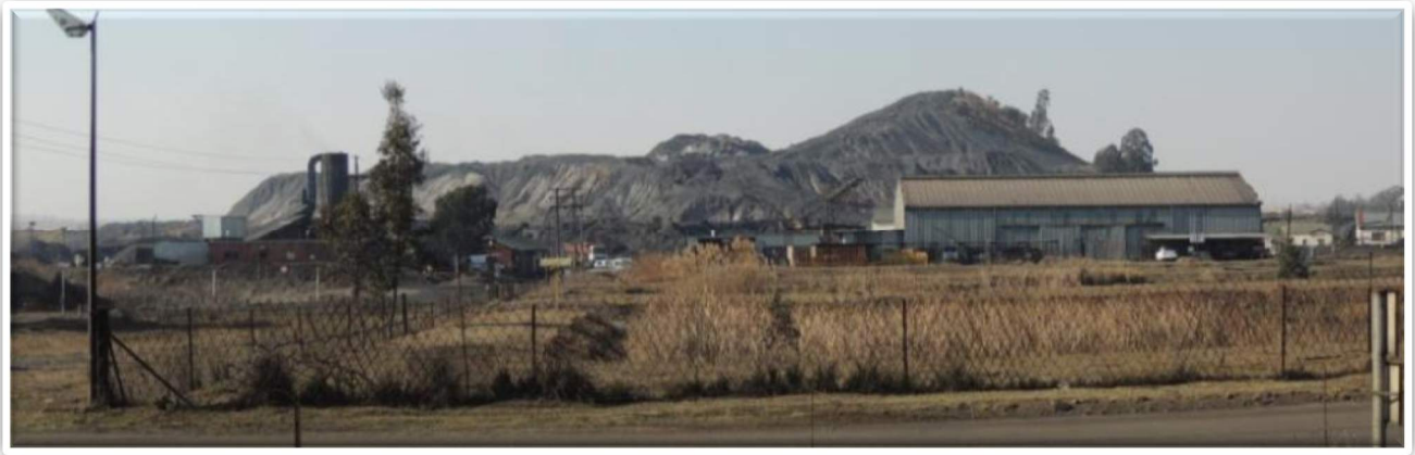
Figure 7: Photograph of existing SA Calcium Carbide Mine site workshop and waste dump
