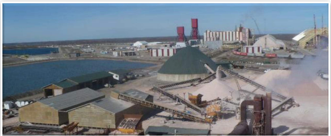
Figure 8: Photograph of additional mining infrastructure, Rocanville mine site, Canada (Source: www.nscminerals.com )
