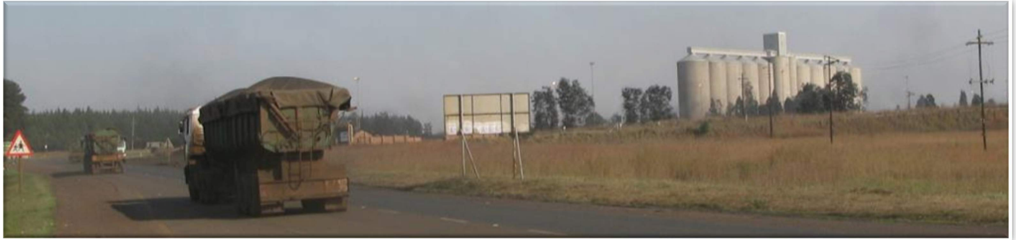
Figure 42: Photograph from R11 towards existing Panbult siding located behind bridge to right of silo.
