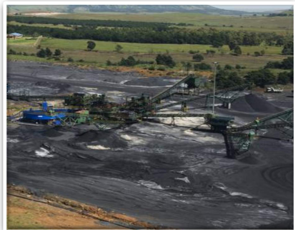
Photograph example of stockpile infrastructure, Kiepersol Colliery, Piet Retief (Source: www.cdn.mg.co.za)
