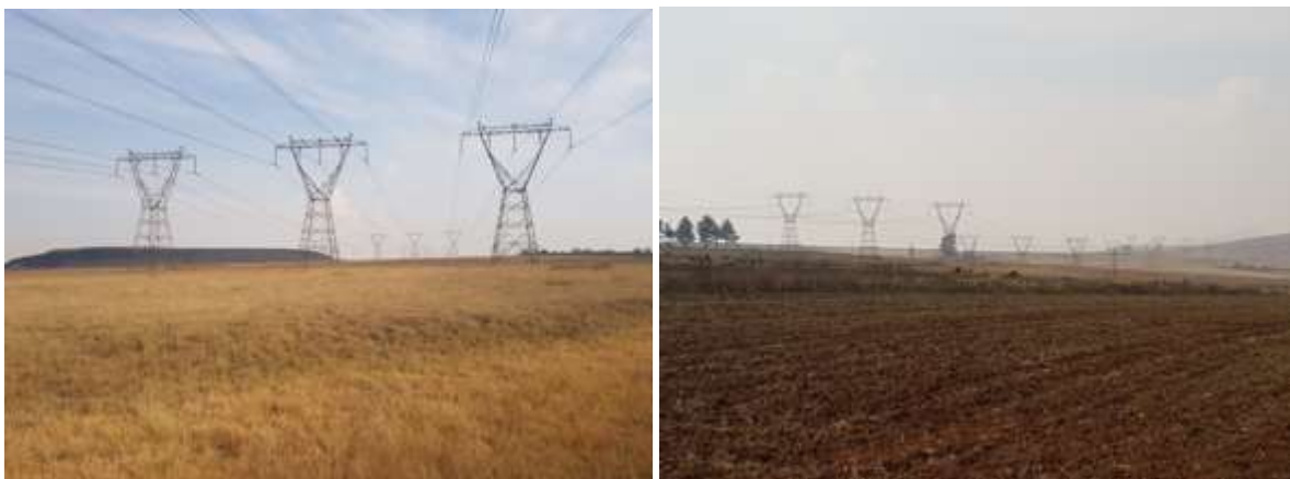
Figure 9- Eskom Transmission Powerlines along proposed Route A conveyor belt
