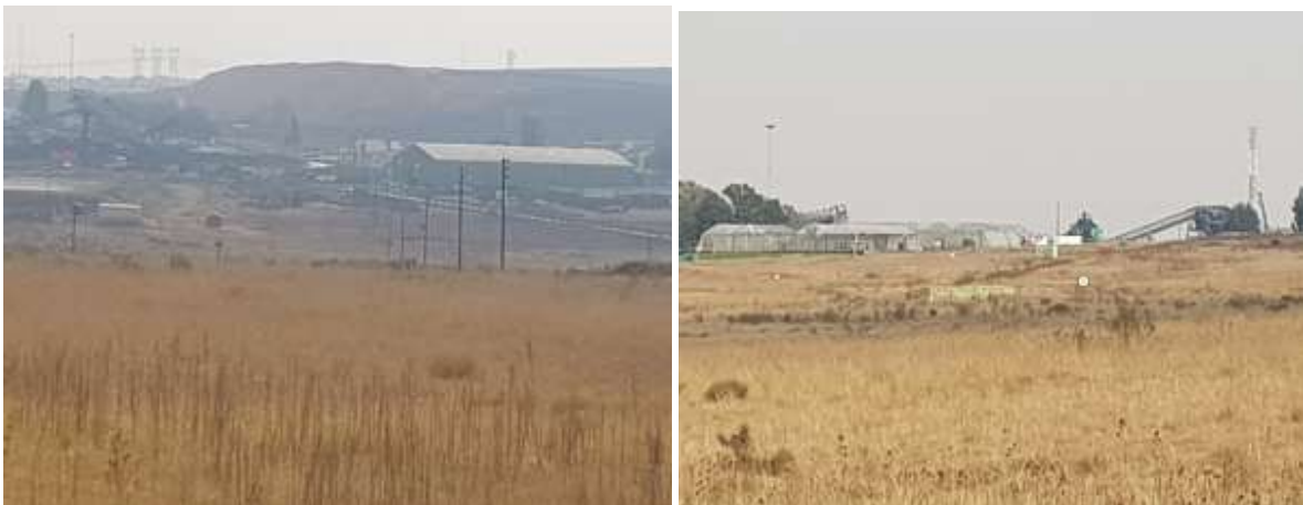
Figure 15-Dorstfontein West mine infrastructure and shaft
