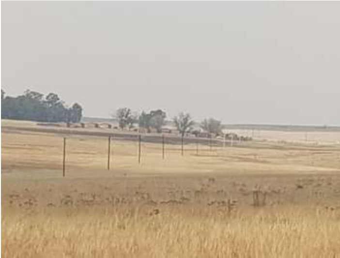
Figure 10- Distribution line to Dorstfontein farm labours compounds.
