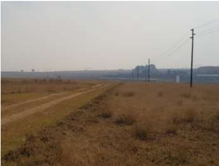
Figure 11- Transmission line to Dorstfontein West shaft and main mine plant
