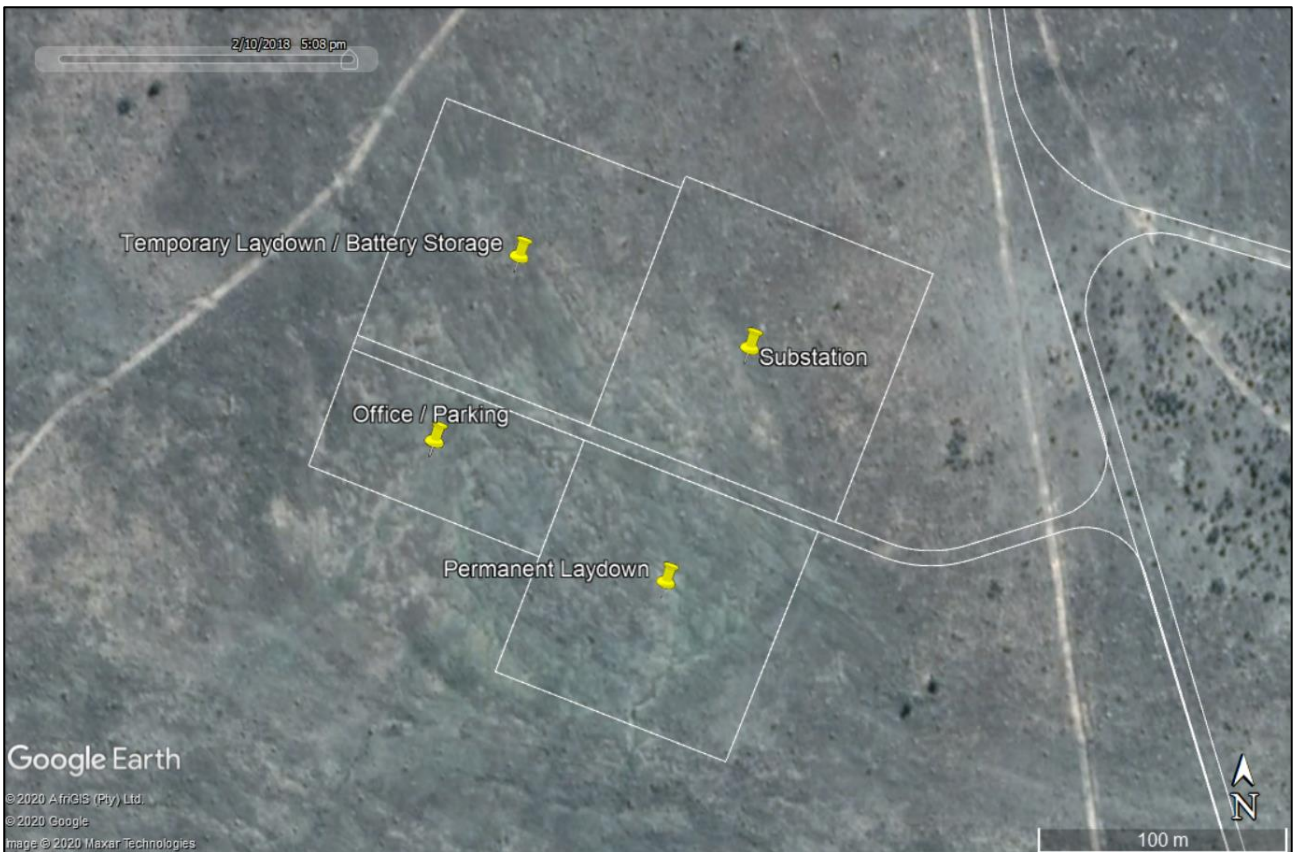
Aerial view of the area in which the substation, offices, laydown areas and BESS would be located.
