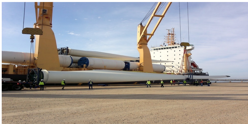
Figure 8: Cranes at Port of Entry
