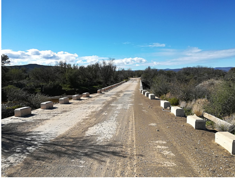
Figure 14: Narrow bridge on DR02249
