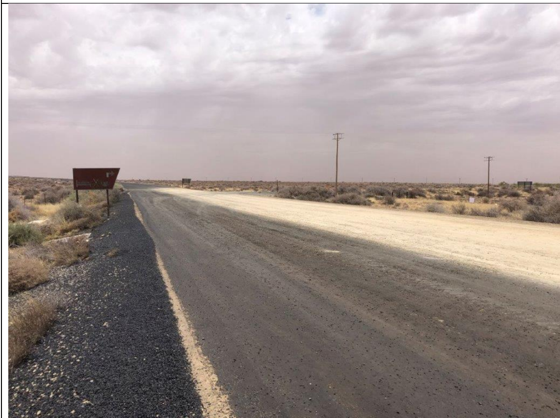
On the boundary fence at the intersection of the road to Copperton and the R357
