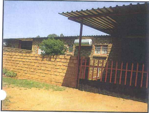
Solar heating of water
