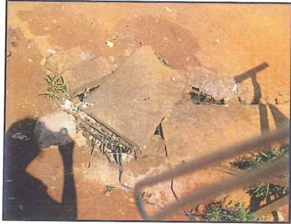
Blocked and insufficient grey water drainage
