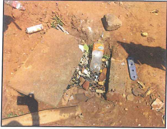
Blocked and insufficient grey water drainage
