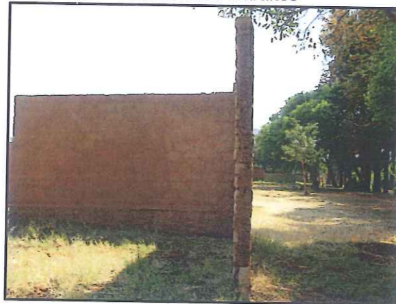
Single brick layer walls
