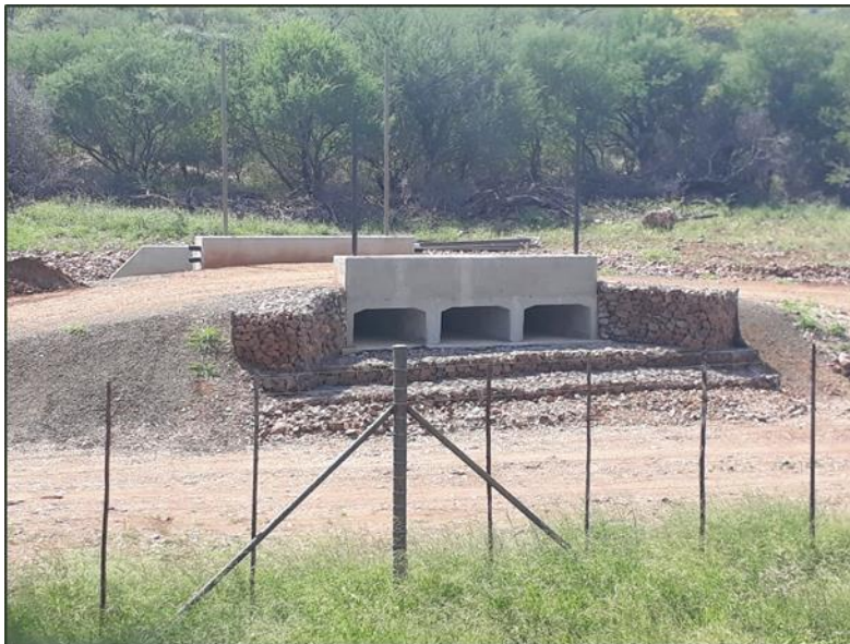
Culverts installed for the patrol Road along the fence
