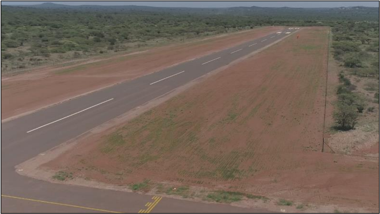
Hydroseeded edges being established
