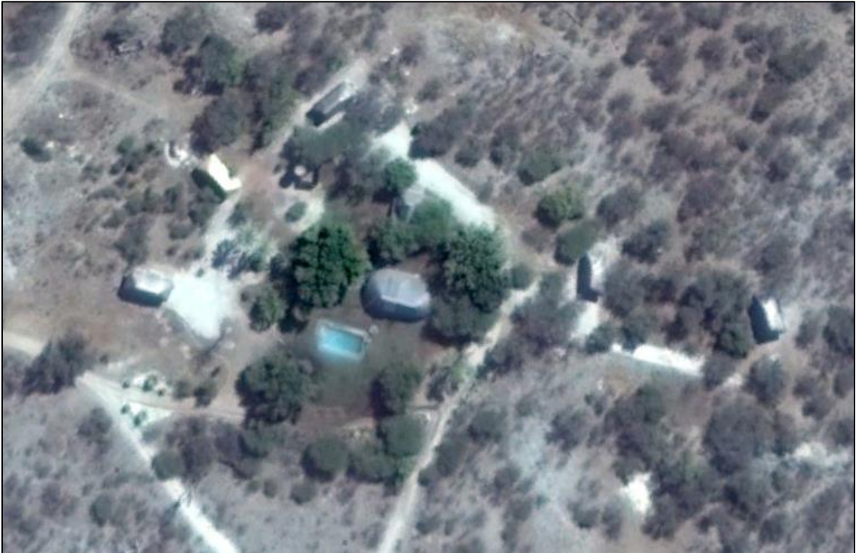
Leadwood Lodge prior to upgrading
