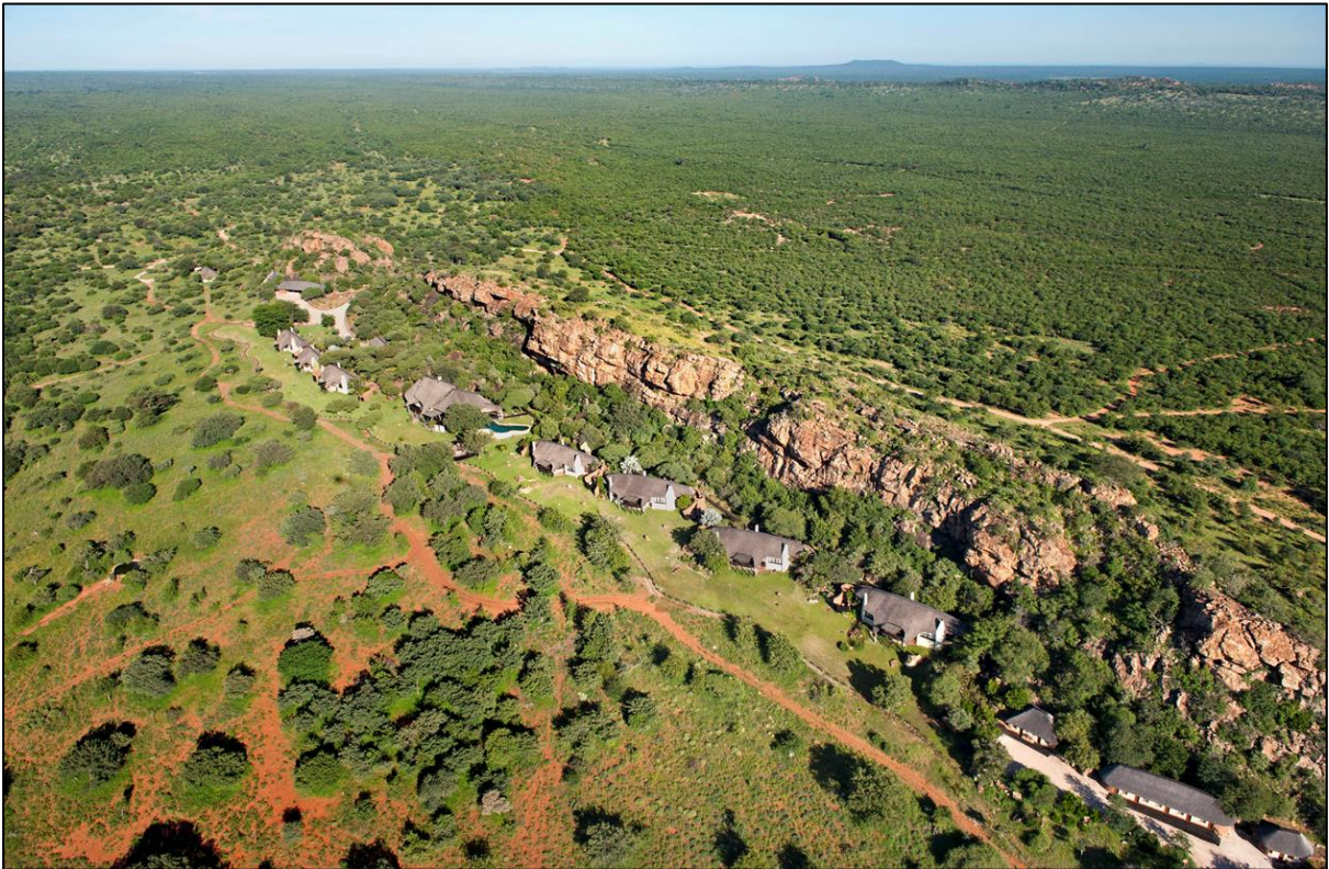
Overview of Main Lodge prior to refurbishment
