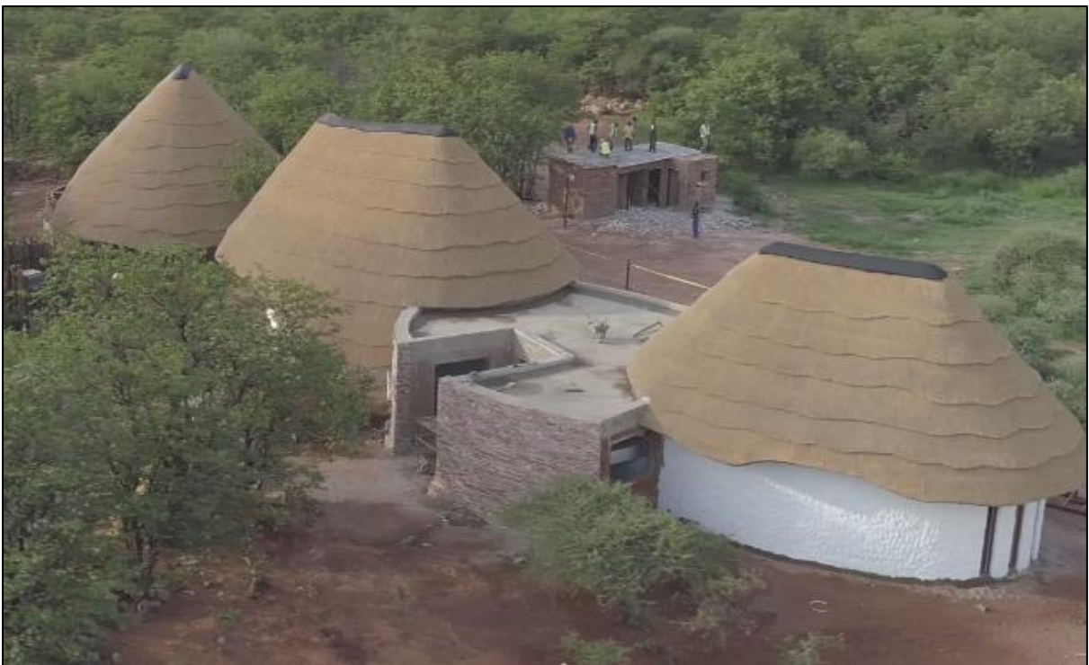
Sulphur Springs Day Spa (back view)
