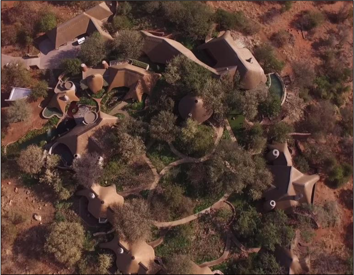
Aerial view of Pienaar Lodge after upgrading
