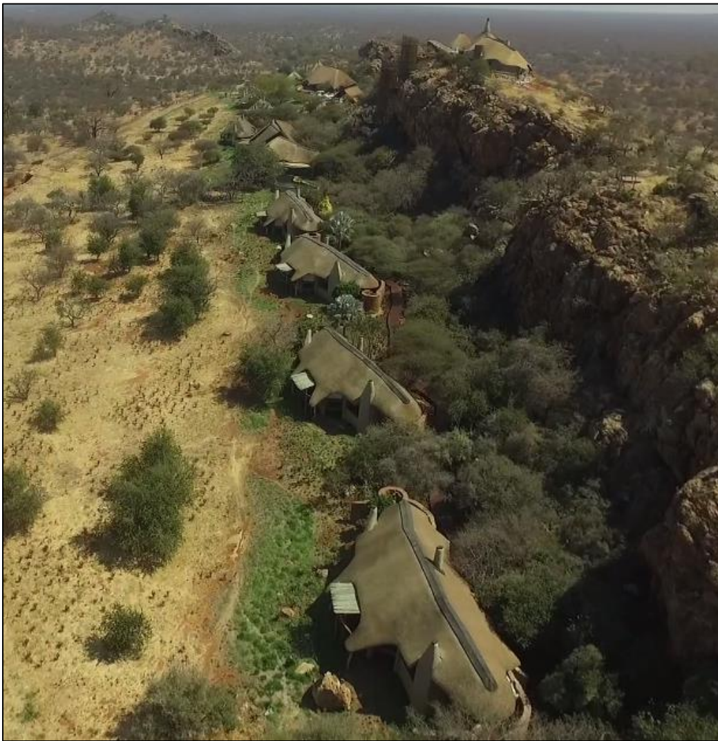
Main Lodge and Presidential Villa viewed from east to west
