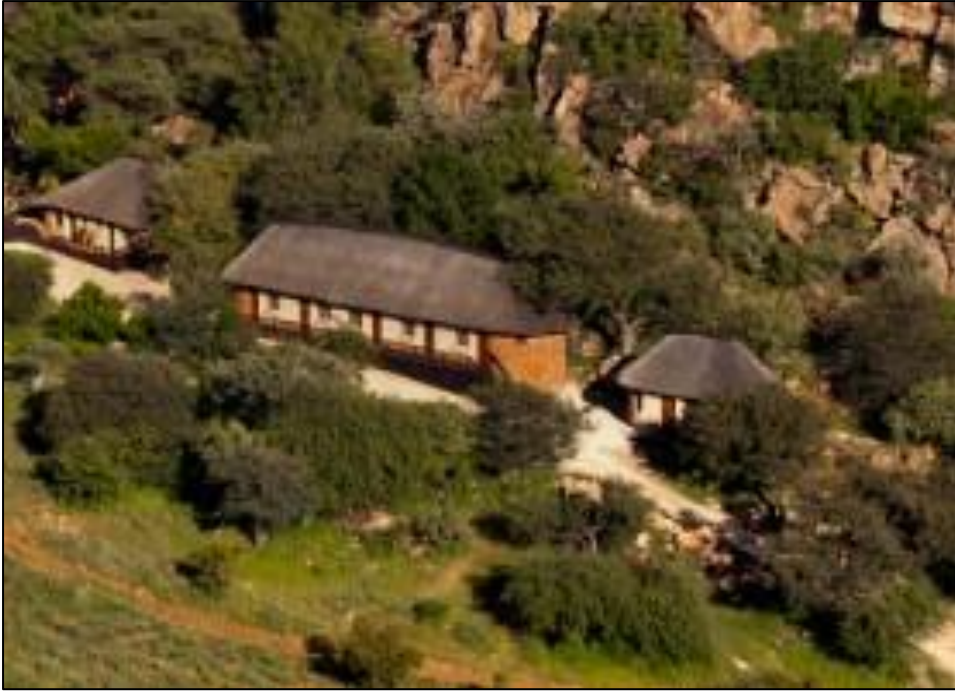
Back of house prior to upgrading
