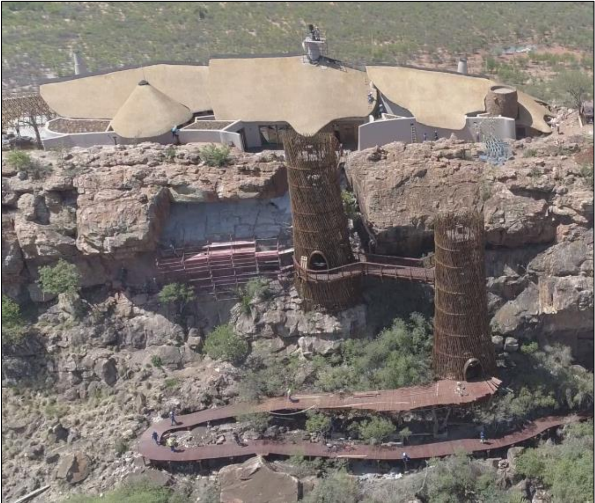
Presidential Villa and lifts to provide access other Villa's
