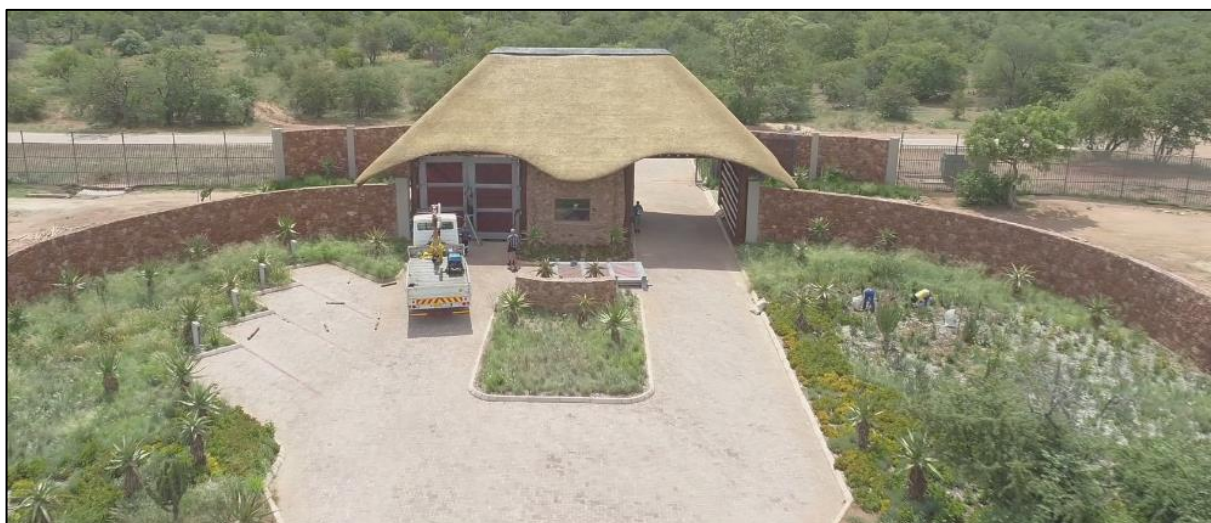
Main Gate along the N1 Highway
