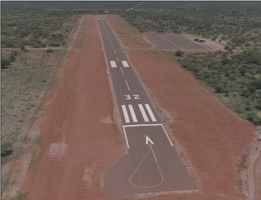
Airstrip after resurfacing and widening
