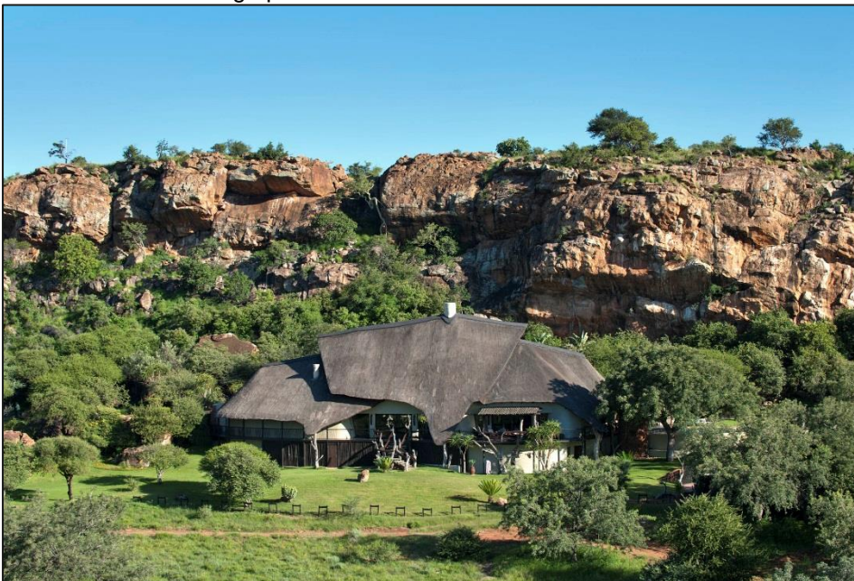
Central Facility prior to upgrading
