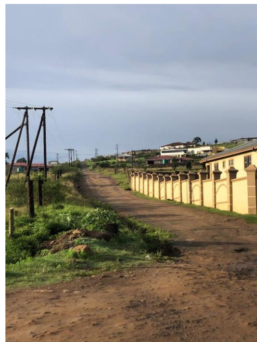
Figure 7: Unnamed Gravel Road South Approach
