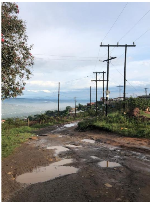
Figure 6: Unnamed Gravel Road North Approach
