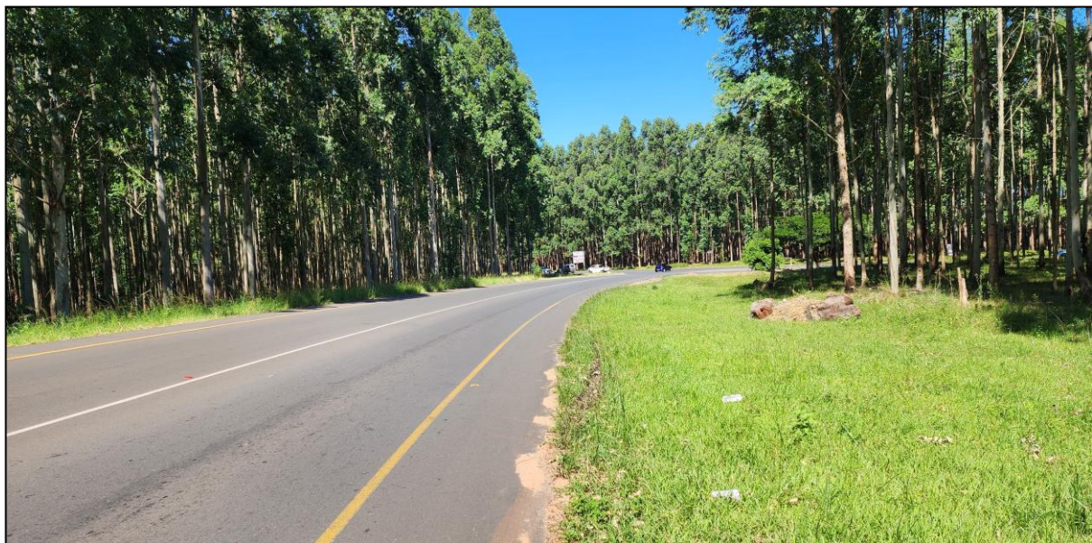
Figure 21: View to the right (south towards P106) from the Development Access Point 1.
