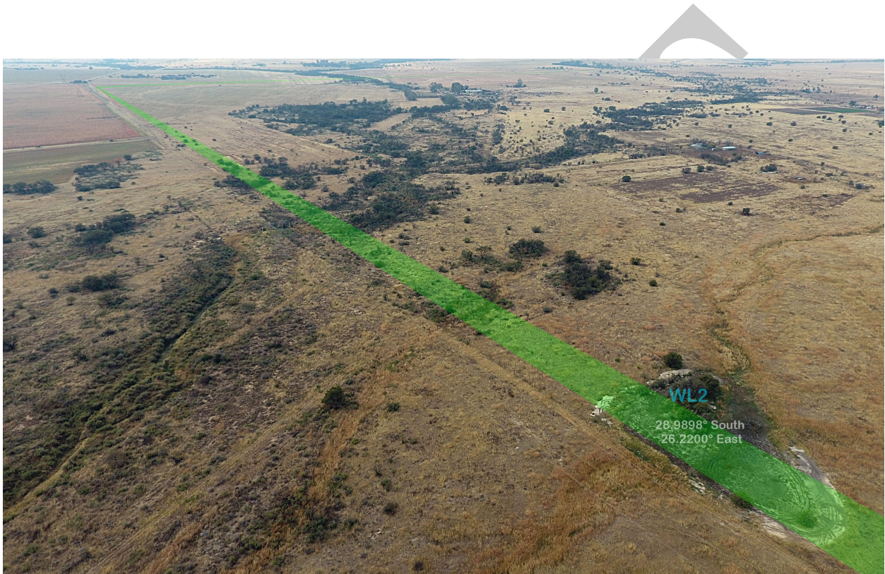
Figure 5: The north-eastern aspect of the proposed main power line (green) where it crosses the eastern branch of Stinkhoutspruit. In its current alignment it goes straight over a prominent wetland (WL2; see Figure 2). Up to the north-eastern (upper left) corner, the line will run parallel to the existing 1HAR/MER power line which runs north (left) of the proposed line. Note the strip of cleared habitat along this existing power line.
