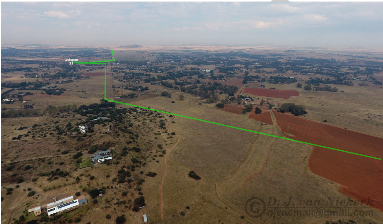
Figure 3: The first part of the proposed power line route (green line) between the proposed Outspan and Rooidam substations illustrating the transformation of Bloemfontein Dry Grassland (Gh 5) into agricultural land and smallholdings. The hill in the foreground-left represents a largely intact isolated patch of Bloemfontein Karroid Shrubland (Gh 7) (Fig. 1).
