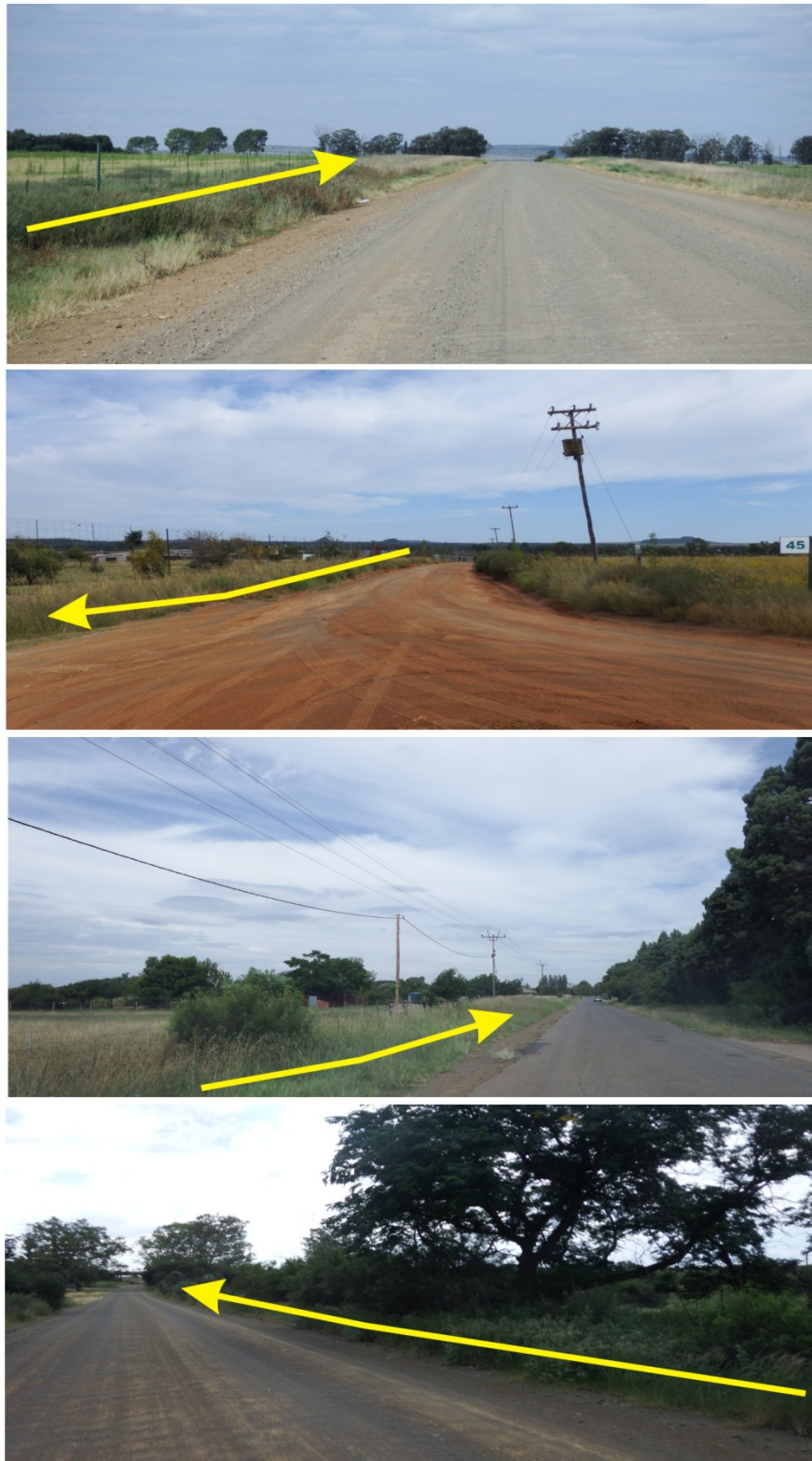
Figure 7. The powerline footprint primarily traverses existing road reserves, degraded farmland and areas formerly disturbed by the residential developments.
