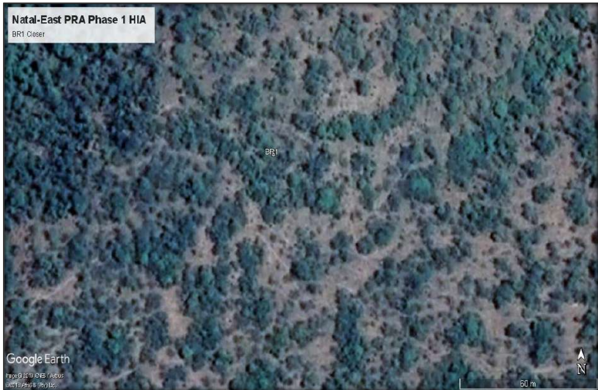
Figure 30: A closer view of the BR1 trench location (Google Earth 2019).
