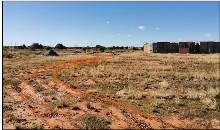
Figure 5 Extreme degradation followed the removal of topsoil. Ground cover represented by pioneering grass species. (Red) tire tracks of construction vehicle adding to the compaction of the soil.
