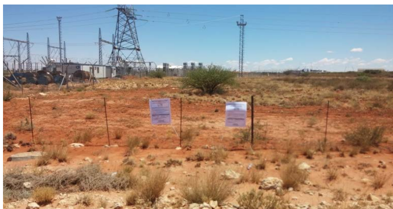
Figure 8: Site notices displayed at the Eskom sub-station near Groblershoop
