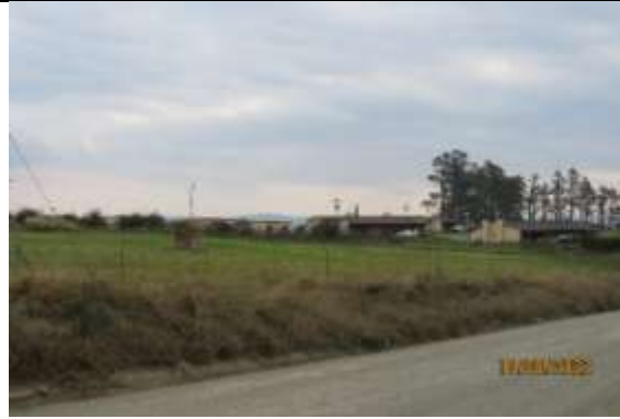
Feedlot staff housing along D73, asbestos roofing scheduled for removal October 2022
