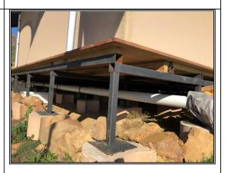
Figure 4 Steel frame and supporting poles underneath office tent
