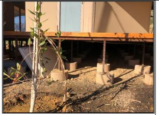
Figure 9 Supporting frame and poles underneath mess tent
