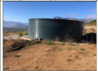
Figure 35 Reservoir on concrete slab
