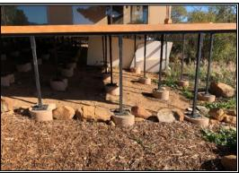
Figure 20 Closer view of platform supporting accommodation tent
