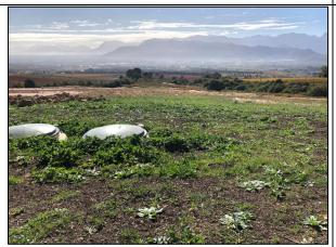
Figure 41 Second pair of bio septic tanks in north-east corner of site and typical state of surrounding pastures
