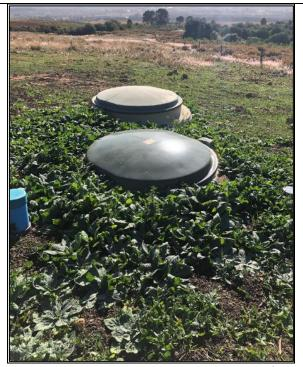
Figure 7 Buried bio-septic tanks in north-east corner of site
