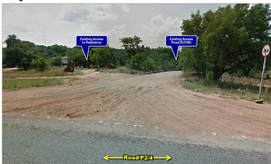
Figure 8: Existing Formal Site Access
