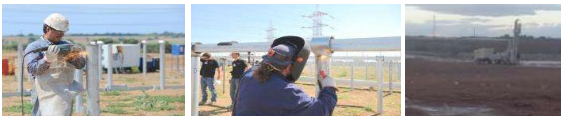
Figure 14: On-site construction of the PV arrays
