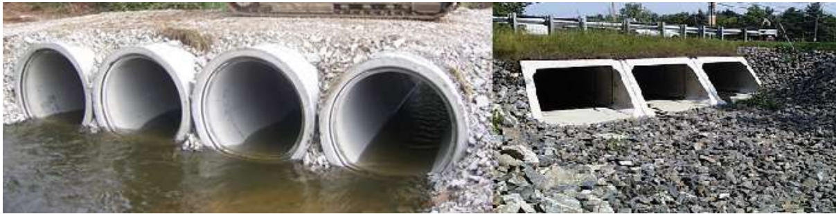
Figure 24 Installed concrete pipes and culverts
