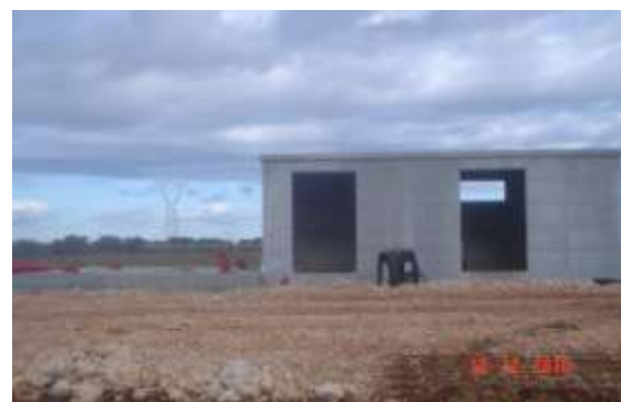
Figure 9: Foundation of a typical on-site building
