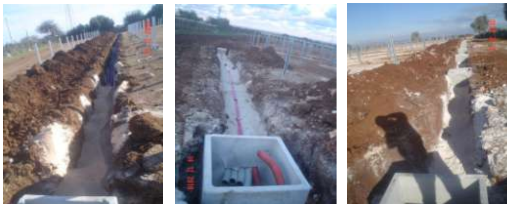
Figure 8: Typical cable trenches
